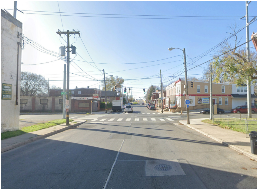
Figure 60: Existing Stop at Heald St and C St
