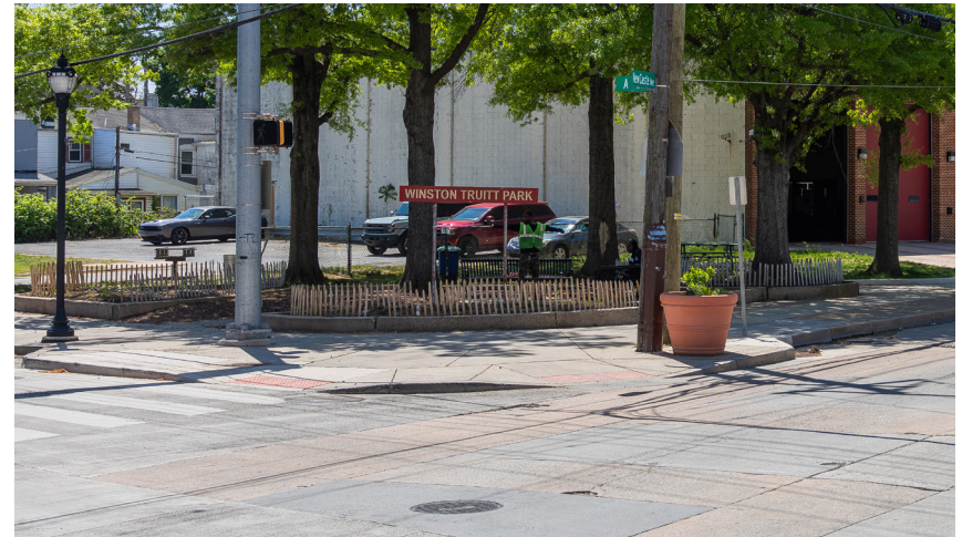
Figure 43: Curb Extension Example in Southbridge
